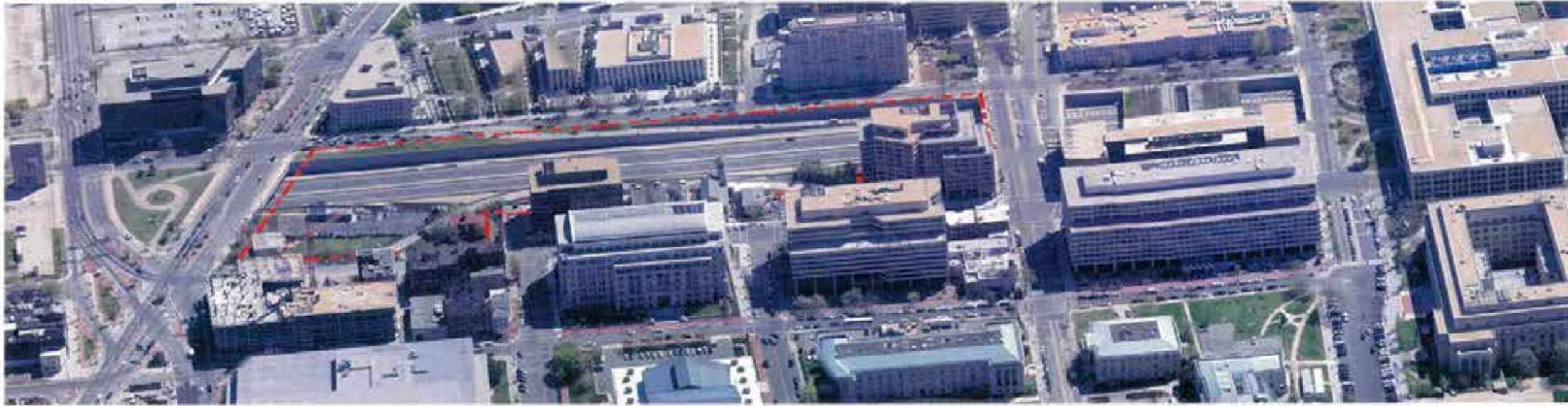
VIEW FROM WEST
