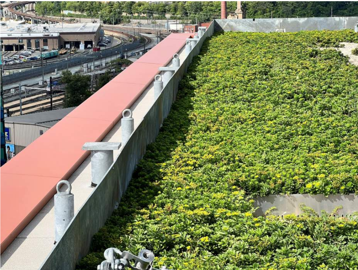
WASH DC - STEEL METAL PLATE
