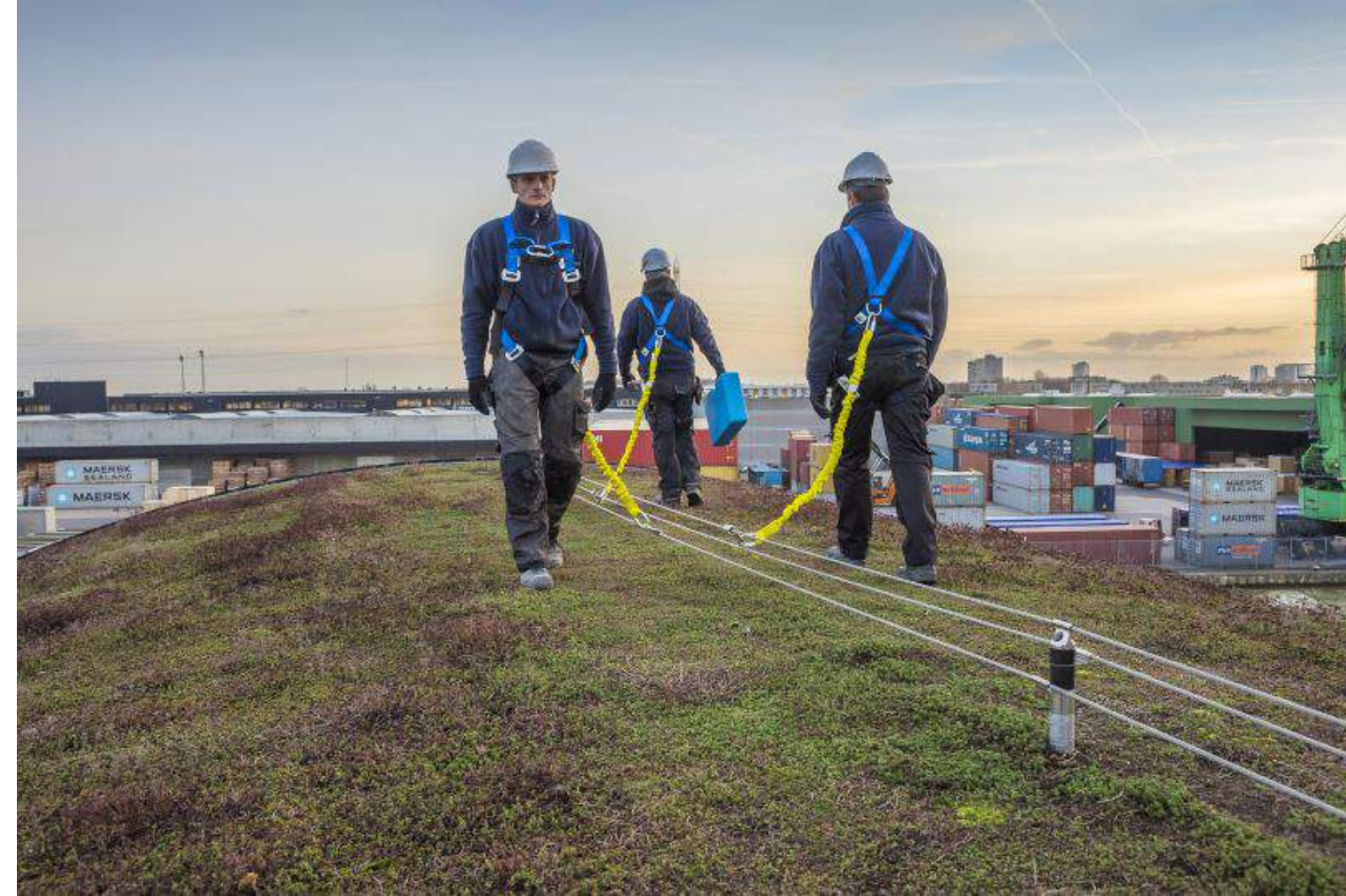
EXAMPLE OF SAFETY TIE BACKS IN USE
