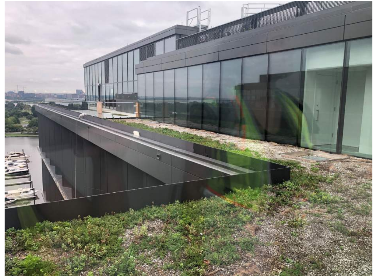
PENDRY HOTEL, WASH DC - COATED METAL PLATE TO MATCH METAL CLADDING
